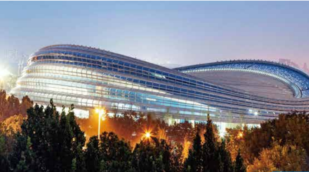
* Beijing Winter Olympics National Speed Skating Pavilion project "Ice Ribbon"
