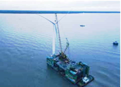
In August 2022, the first hoisting of Vietnam's Ca Mau 350MW offshore project was completed, which is the largest offshore wind project under construction in Southeast Asia.
