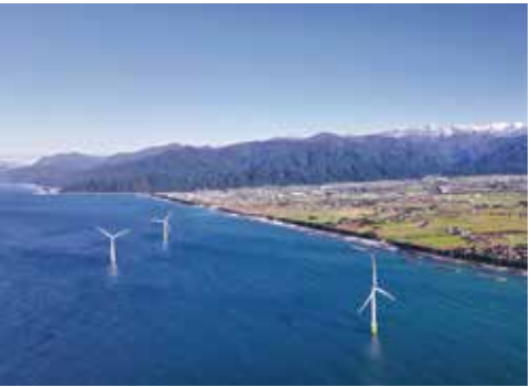
In October 2023, the Nyuzen offshore wind project in Nyuzen Machi, Japan, which was the first to use the Chinese offshore wind turbine, was completed and put into operation.
